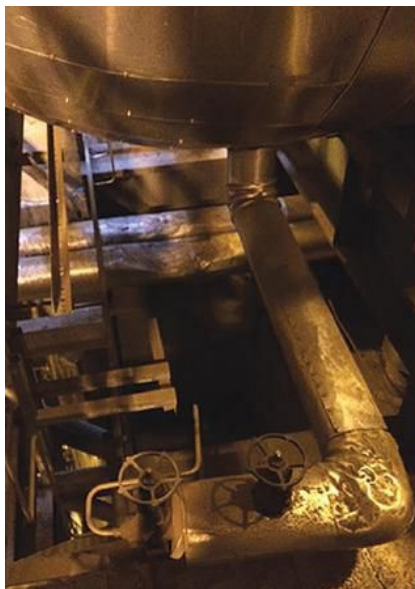
Figure 5. Lower connection tubing on a differential pressure transmitter.
