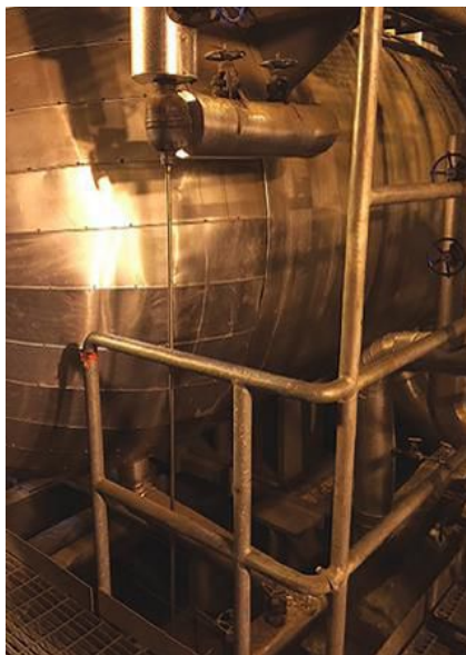
Figure 4. Upper connection tubing on a differential pressure transmitter.
