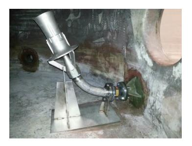
Because of the unique design of the TLA, for every one gallon pumped through the nozzle, the TLA will entrain four gallons, meaning that a total of 5 gallons will be moved for the cost of pumping one. The fluid pumped will generate an effective flow field in the tank which varies depending on the pump pressure and flow. As the flow field increase in length, the diameter of the flow field increases as well, ensuring that there is movement in the tank.
